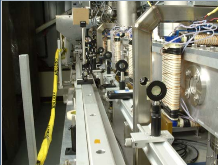
Outside Undulator Box with FEL Optical Transport Line
